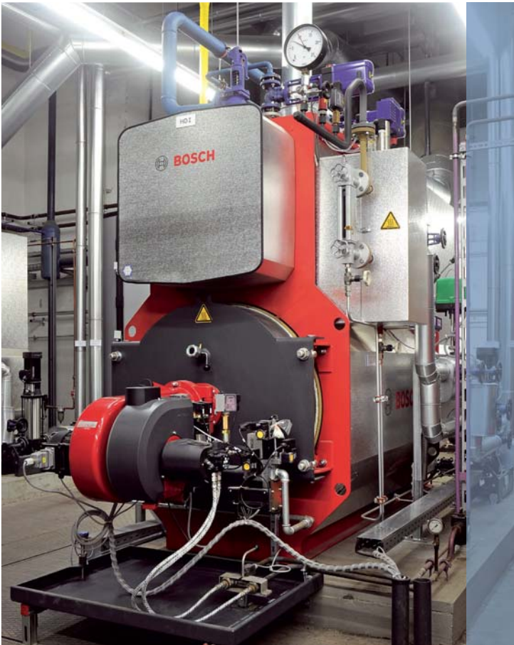
The compact steam boiler U-MB with economizer and fired with natural gas.
