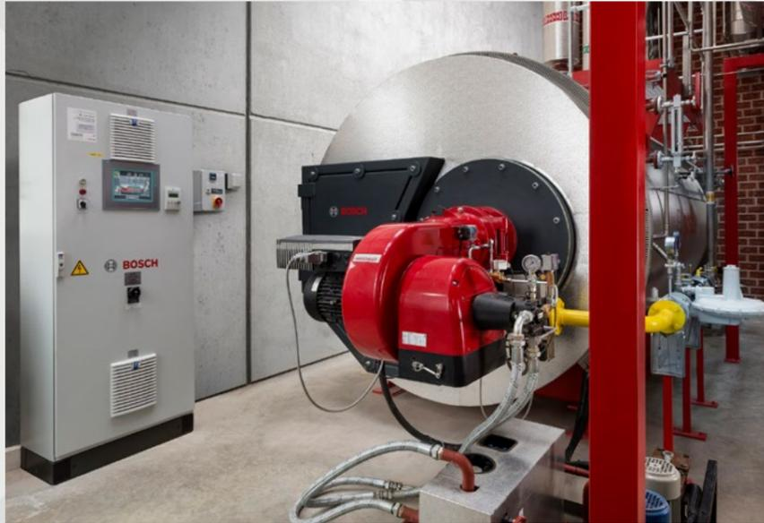
The intuitive, PLC-based boiler control BCO offers a very high level of operating data transparency for optimum boiler operation.
