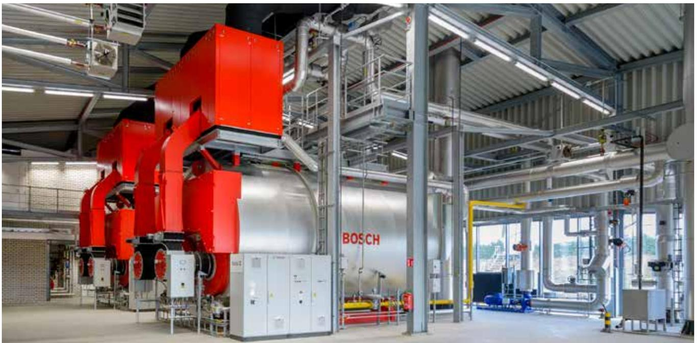
The NO<sub>x</sub> values are under 50 mg/Nm<sup>3</sup> at the customised boiler system in the Pieter Wiersma heating plant.
